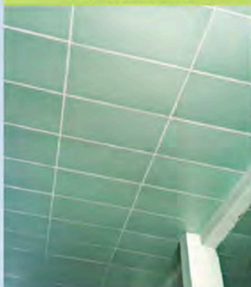
Under deck Insulation
